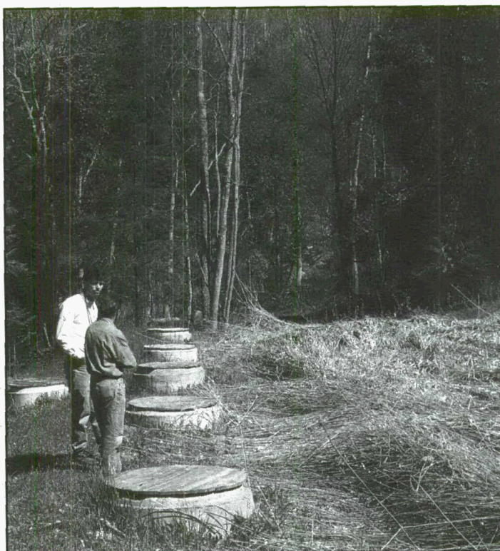
An artificial wetland used for hotel wastewater treatment. Lac Simon, Quebec.
