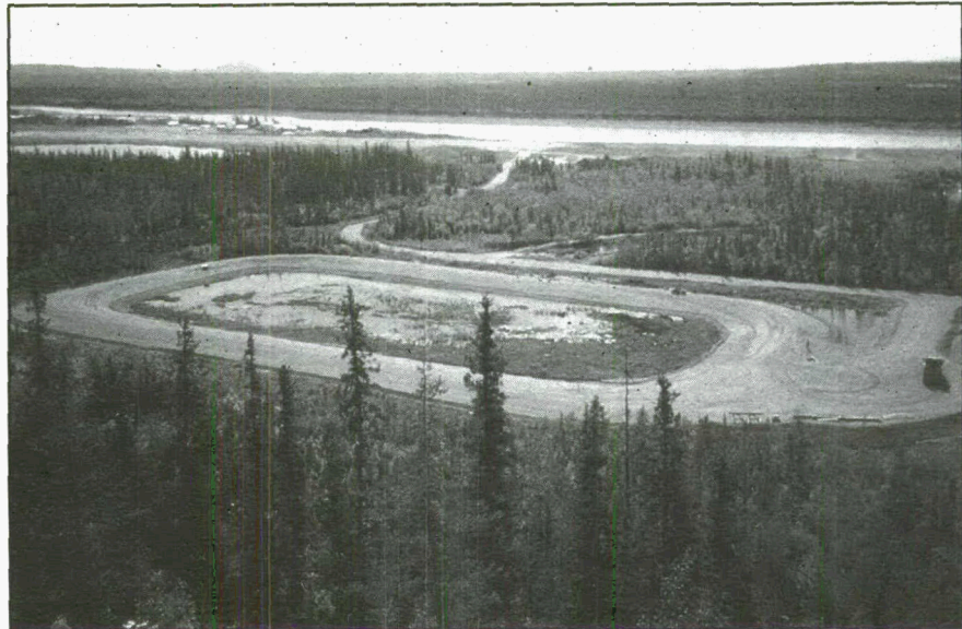
Municipal wastewater lagoon and seasonal discharge wetland. Old Crow, Yukon.
